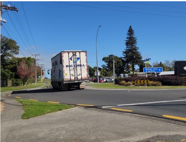
Figure 18: Areas of circulation lane not being used by vehicles
