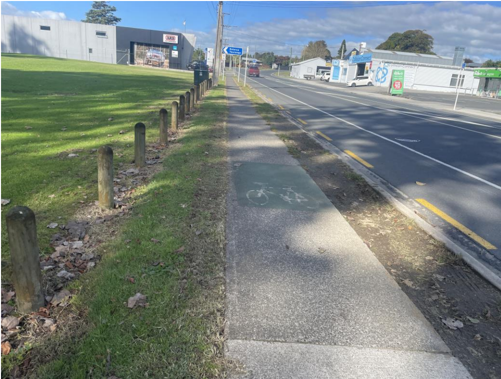
Figure 1: Existing cycle path marking on northern footpath of Cook Street
