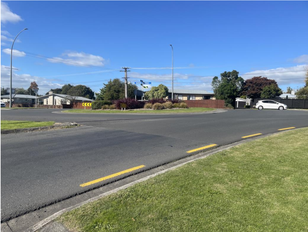
Figure 14: View of Roundabout (Photo taken from Cook Street)
