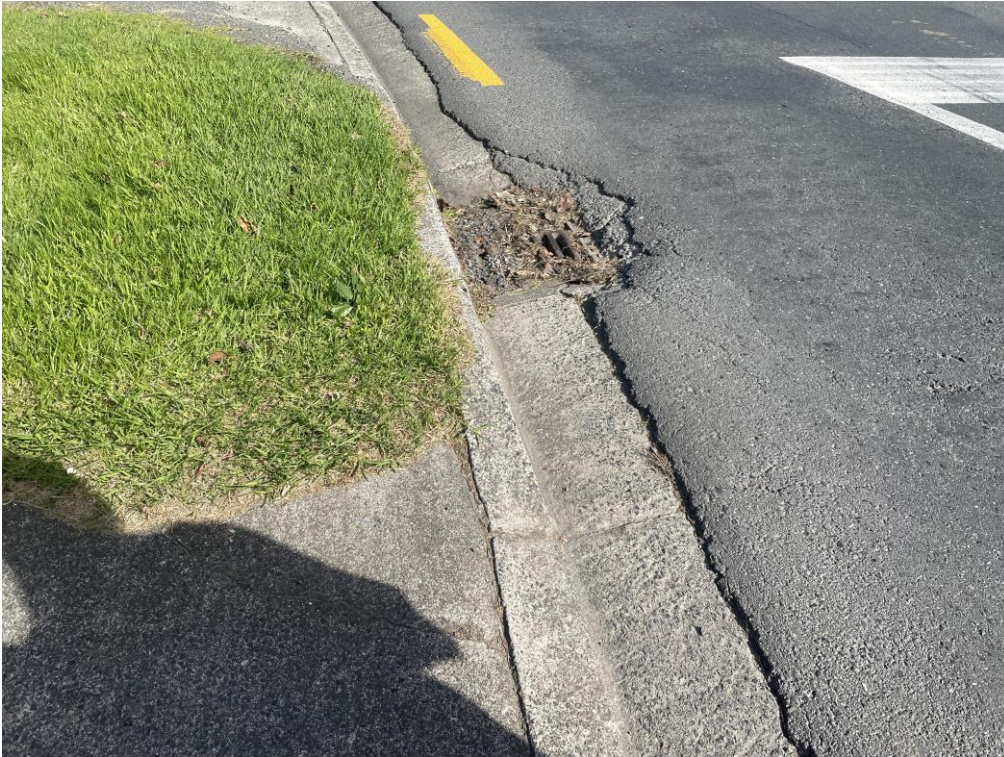
Figure 11: Blocked catchpit
