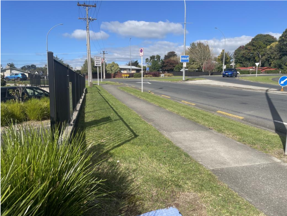
Figure 5: 'Heavy Vehicle Route' sign indicate high volume of heavy commercial vehicles
